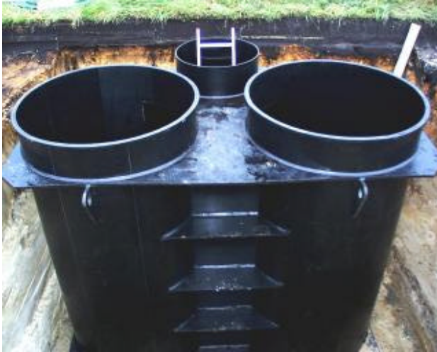
Implanting the 2-fouled station in prepared excavation
