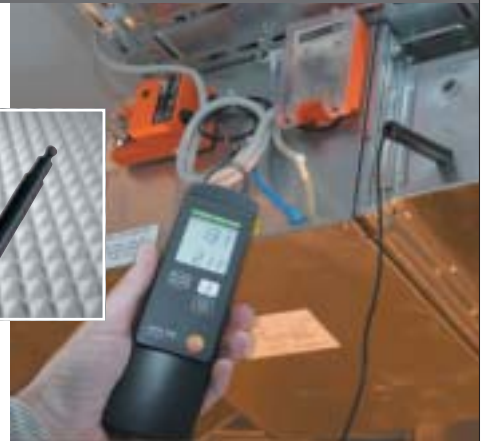
Checking air flow in air conditioning ducts
