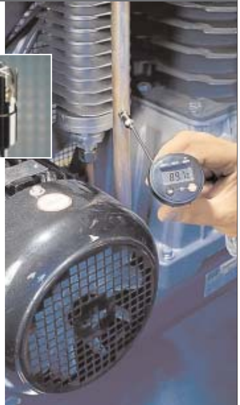
Temperature monitoring in a refrigeration system
