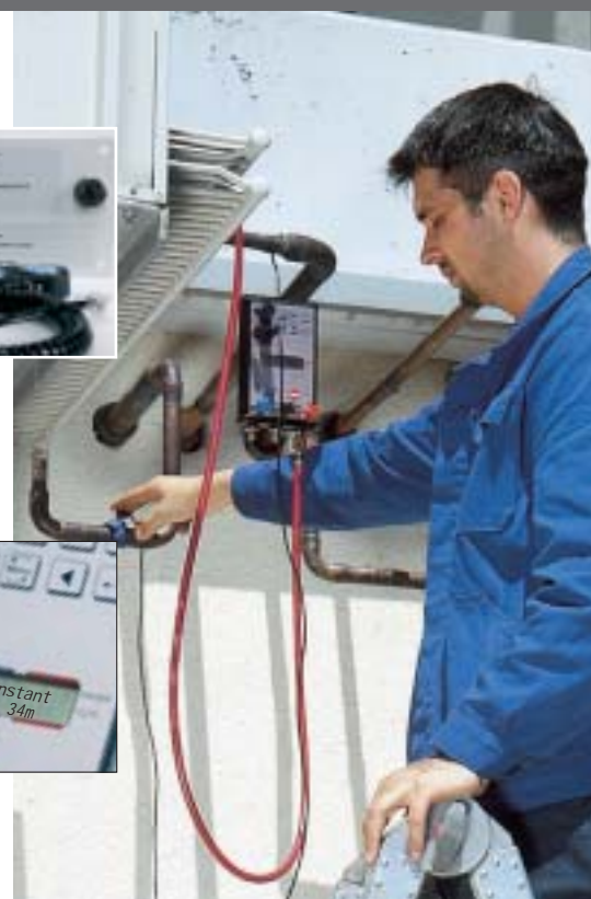
Measuring subcooling using an attached pipe wrap probe
